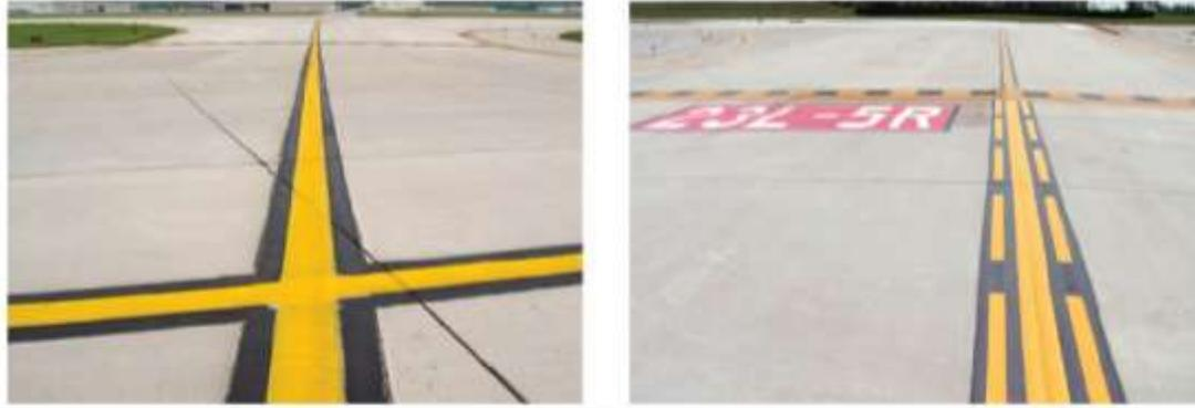
**Figure 2. Enhanced Taxiway Centerline Markings (FAA 2009)**
